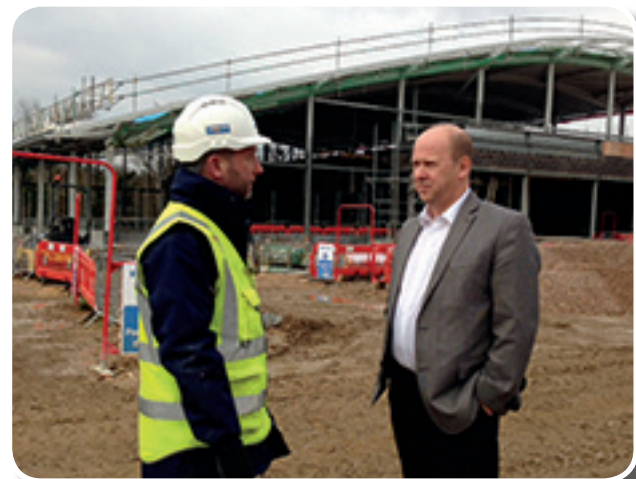
Simon is shown progress on the new £9m Holly Hill Leisure Centre by Balfour Beatty site manager Wayne Smith.
