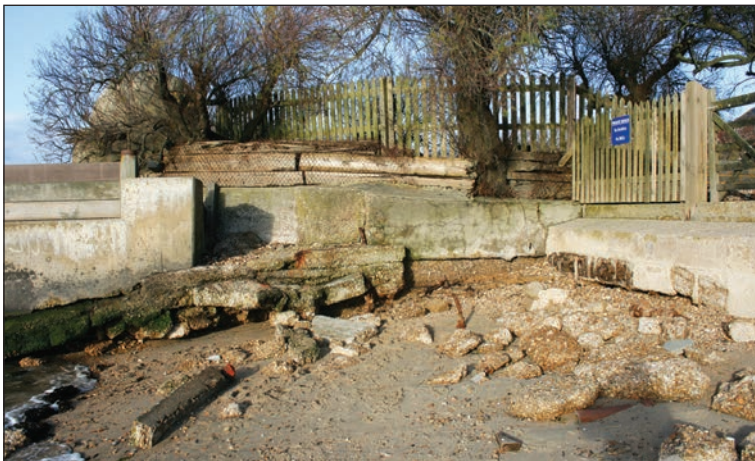
Battered by the sea: Concrete foundations (left) exposed and (above) old groynes have reappeared, almost blocking the beach.
