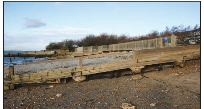
Battered by the sea: Concrete foundations (left) exposed and (above) old groynes have reappeared, almost blocking the beach.
