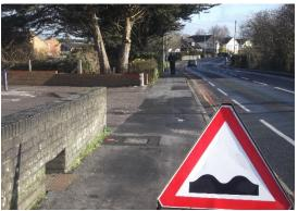
You will have noticed that the road surface in Highlands Road near the entrance to the old railway line is sinking. This is where the old railway bridge was. It was filled in and now the filling has begun to settle. Hampshire Highways are undertaking a geological survey to see how best to solve the problem, as just putting more tarmac on will have little long term effect.
